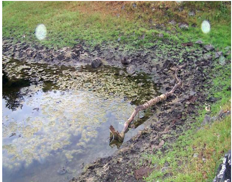
Pond damage and contamination on Hayfield Rd. Trail
