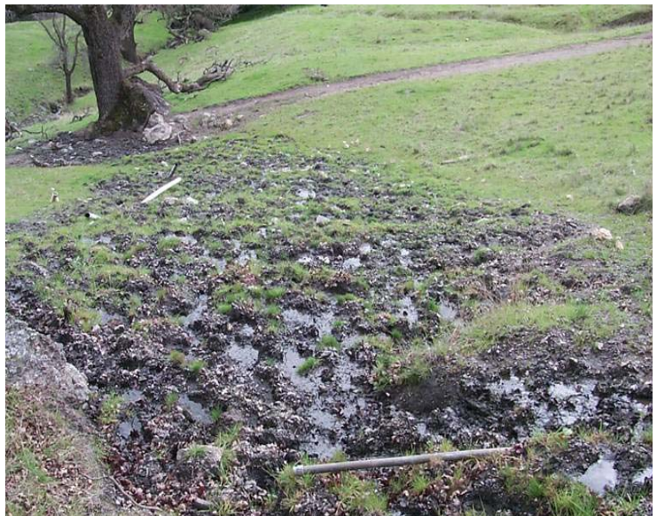
Wetland seep damage on McCorkle Trail
